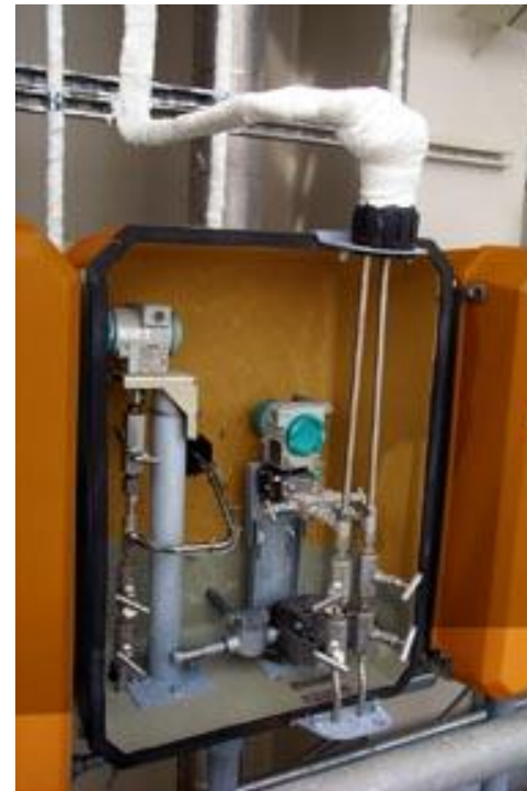
EXPOSED INSULATION
