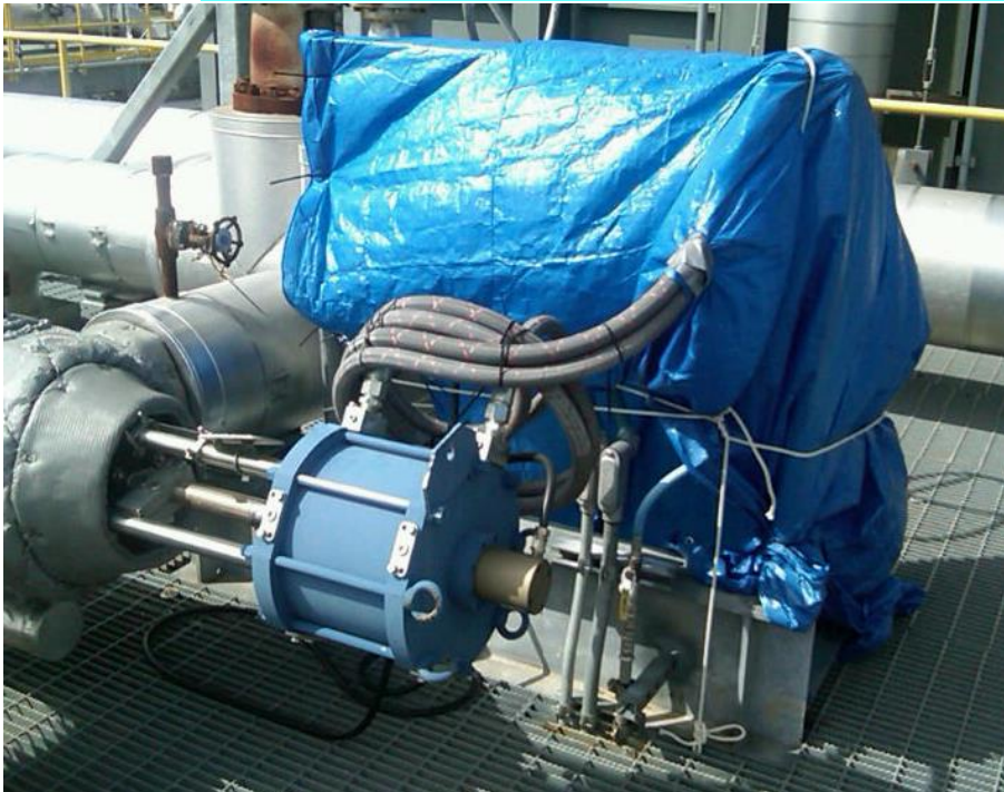
Typical condition prior to freeze protection upgrade
