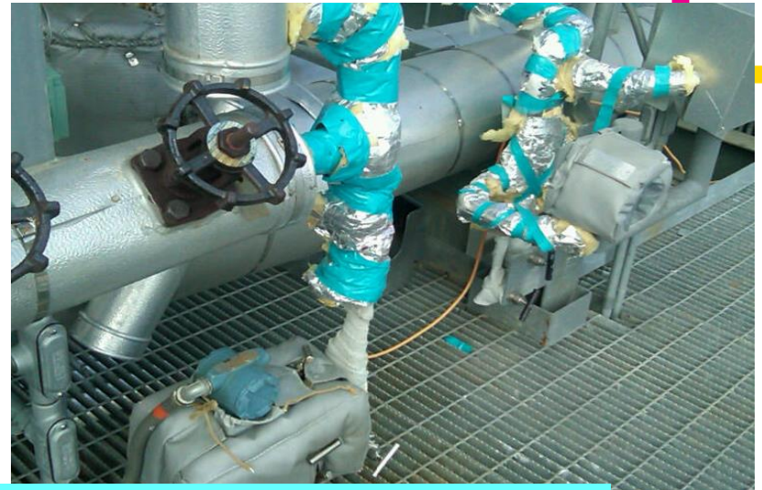
Typical condition prior to freeze protection upgrade
